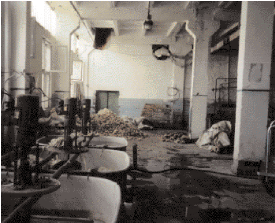
A scouring room in Yerevan
